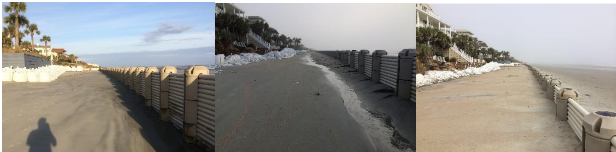
Figure 21. Significant accretion through the WDS during the 2 nd quarter. The figures from left to right are dated 11-30-15, 12-8-15, and 12-24-15.
