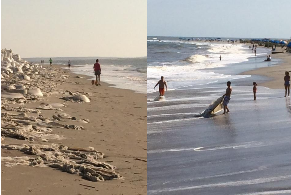
Figure 35. Deteriorated/buried sandbags and individuals pulling sandbags from the surf.
