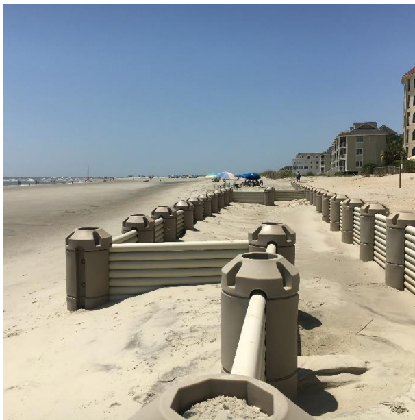
Figure 17. Seascapes performance at end of July 2016 (picture taken 7/30/16). Note significant accretion.
