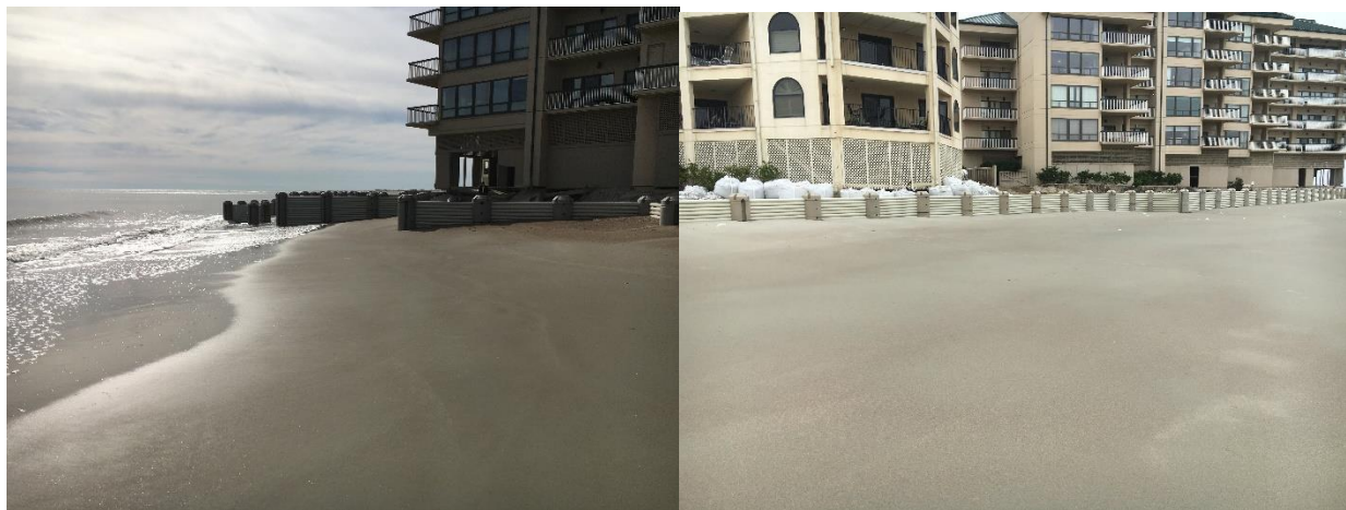
Figure 10. OC north extension (1-14-16) and Seascape during installation yet prior to 3 rd tier completion (1-9-16).
