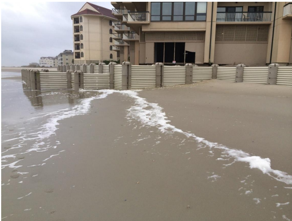
Figure 8. 2 nd quarter configuration on site (with all proposed modifications except full extension to the property line as necessitated by the lowering beach; photo taken: 11/19/15).
