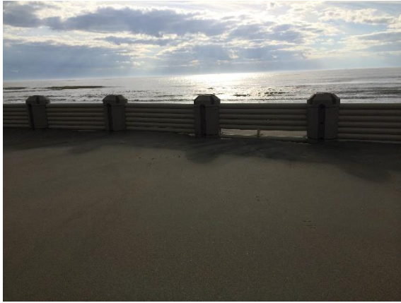
Figure 22. Typical opening used as Beachwood East.
