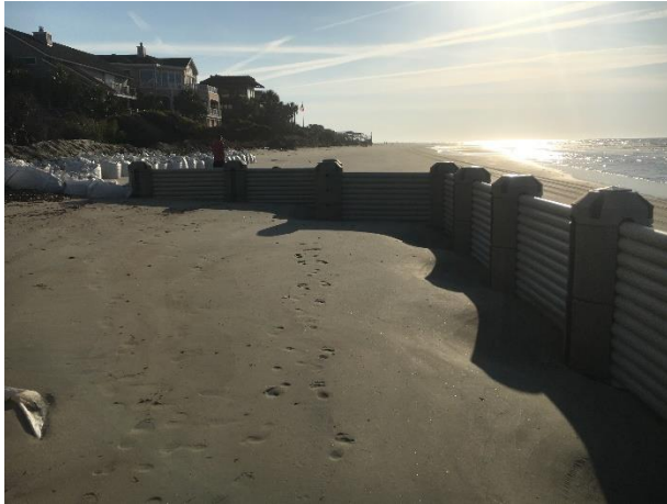
Figure 23. Sandbag extension on north end to allow for access to sandbags behind the WDS and provide closure to sea turtle access.
