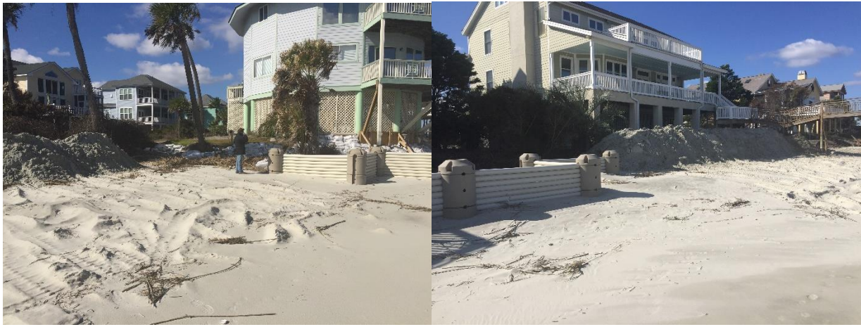
Figure 33. Typical scraping adjacent to WDS (February 5, 2016).
