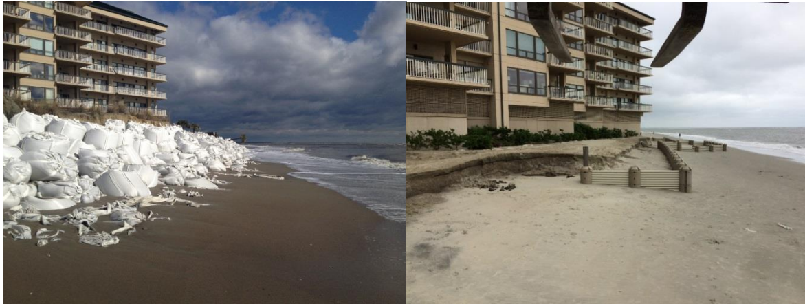
Figure 34. Sandbags and WDS providing erosion and building foundation protection.
